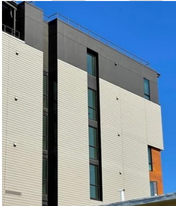
Figure 10. Windows within a recess
